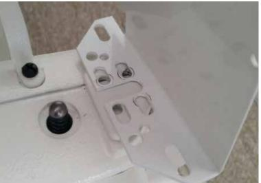
Attach the display bracket to the machine using the screws removed in step 2
